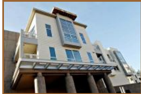
Exterior of Unit #308 (center) that goes for a cool million dollars at Mercer Condos in downtown...
